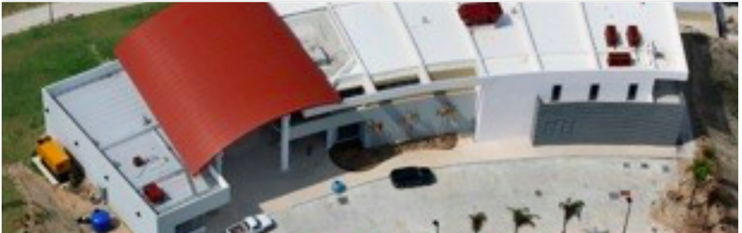
HIGH SCHOOL ROOF USED TO COLLECT WATER
