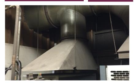
Heat recovery off the 2–50HP compressors was added to add MUA and heat to the plant in winter. Both compressors were integrated in the system which also controls room temps to a min of 40F and automatically uses the heat when temps drop below 50F outside.
