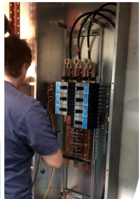
NEW DATA TRUNK BEING INSTALLED
