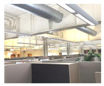
LED lighting was used to upgrade the entire facility and reduce maintenance costs. These uplights had a new fixture insert that was also dimmable for maximum versatility and savings.
