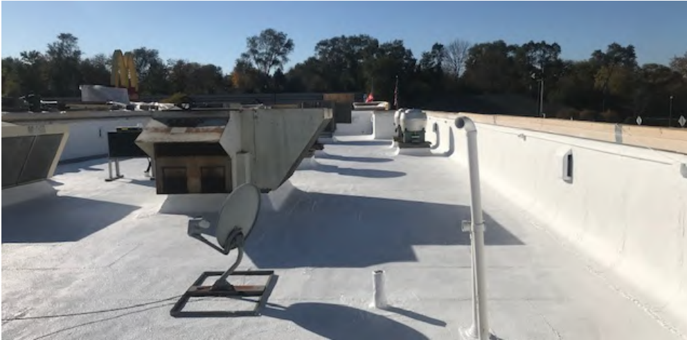
Roof is Restored Using a Renewable ( Sustainable ) Roof System by Adurel
