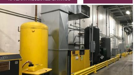
Heat recovery off the 2–50HP compressors was controlled by the new automation to not overheat the aisles next to the refrigerated production. With the lower setpoint and destratification in place the compressor or lights and not almost completely heating the spaces next to the production areas.
